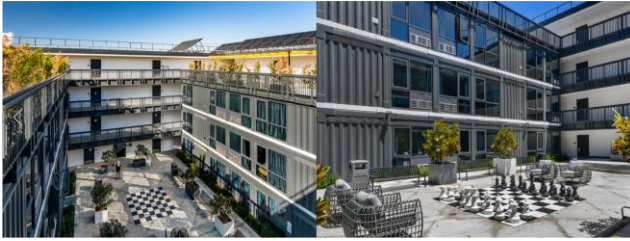
The apartment building's central courtyard (image source: https://ktgy.com/people/mark-oberholzer/ )
