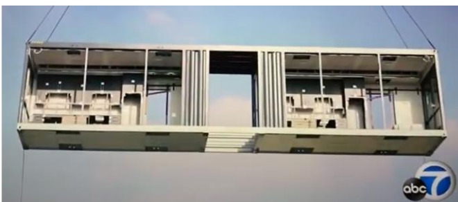
Prefabricated module fully equipped with kitchen and bathroom features (image source: abc-7 News, https://www.youtube.com/watch?v=Vms-lkRbYbk )
