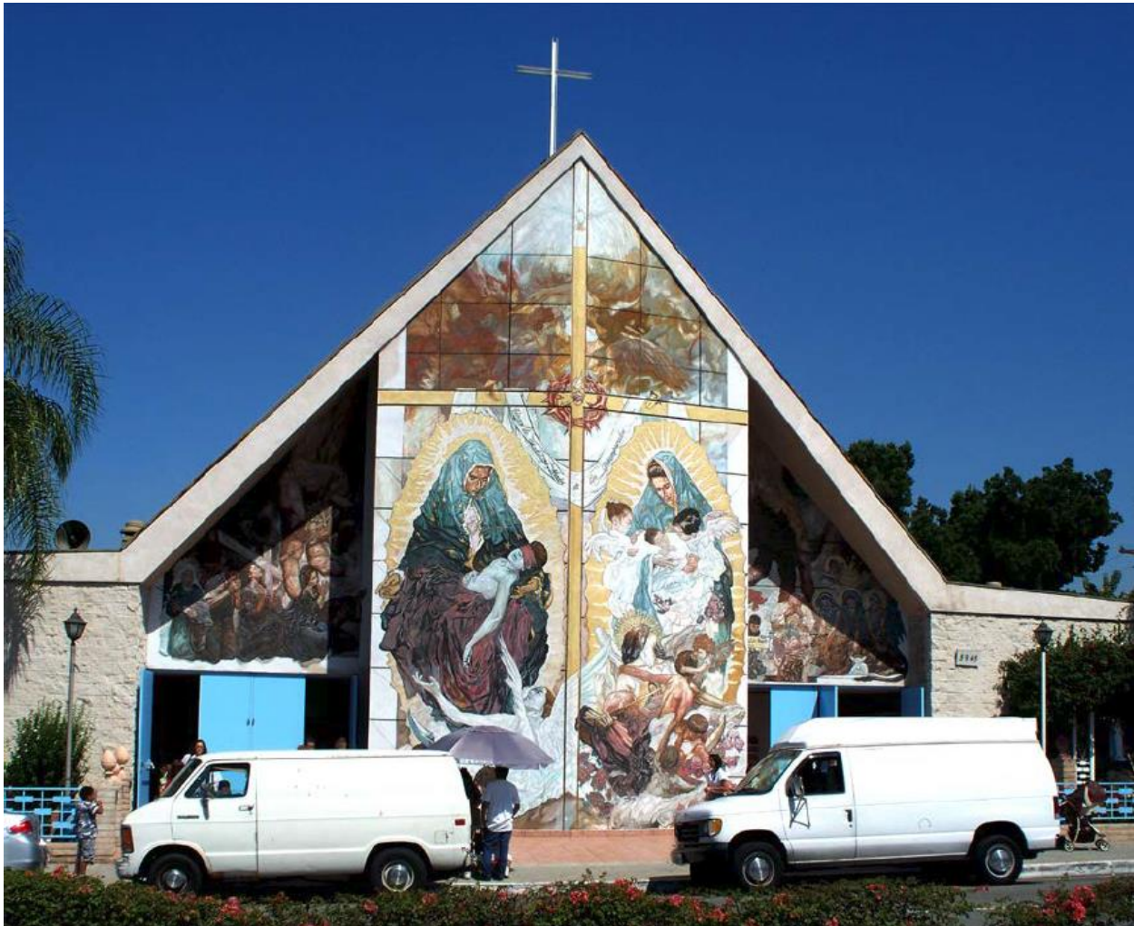
Figures 1. Traditional style mural at the façade of a Catholic Church in Monterey Park.
